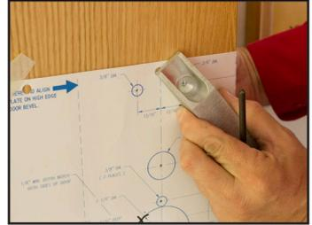
2. Hand tighten the drill bushing screw on the other side of the door. Let the tool rest on the edge of the door as shown.
